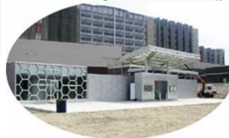
Hydrogen Station in Hydrogen Campus of Kyushu University
